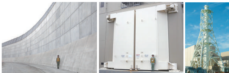
Tsunami protection wall
