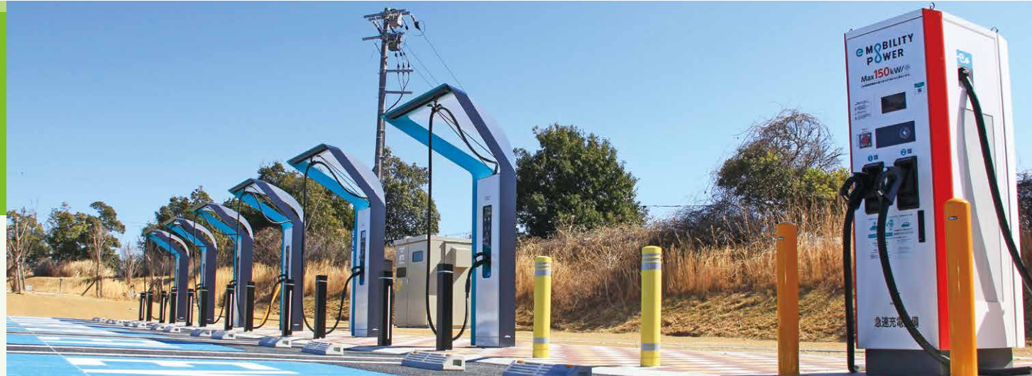
Quick EV charging stands installed in the Hamamatsu Service Area (on the outbound roadside)
