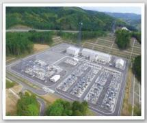
Hida Converter Station connecting a 50Hz area (eastern Japan) and a 60Hz area (western Japan) starts operation (March 2021)
