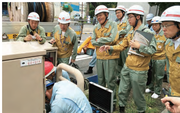
On-site inspection of exchanging work of padmounted transformer
