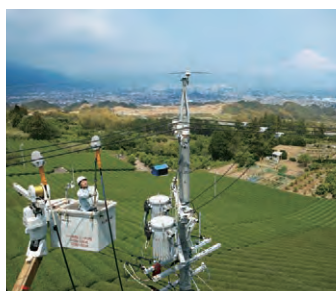
Installation work of distribution lines
