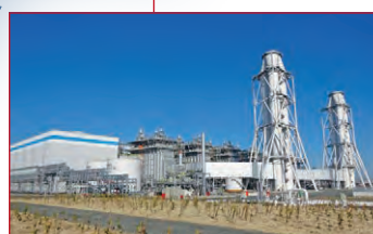
Nishi-Nagoya Thermal Power Station 2,376.4 million kW Highest thermal efficiency in the world (63.08%)**
