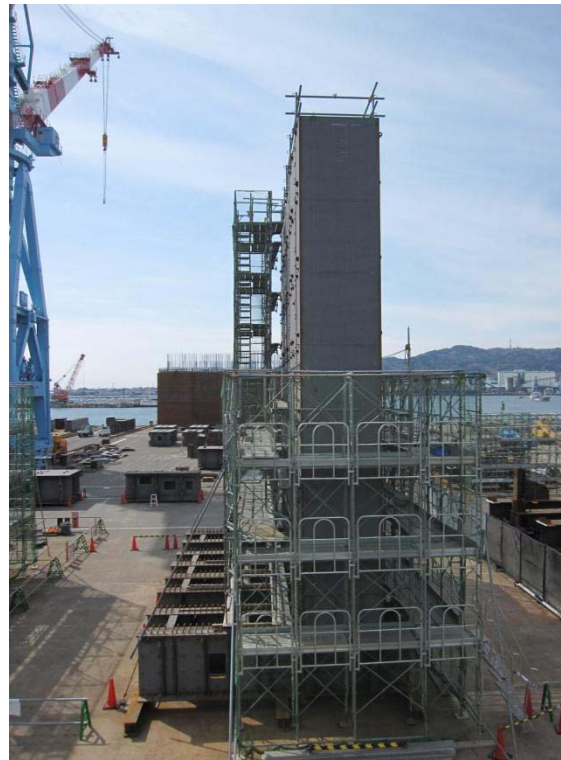
Panoramic photo of wall portion (floor slab and vertical wall) temporarily assembled (1 block)
