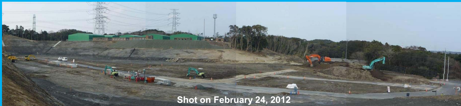
Preparation work of the high ground for the station site (T.P.+40 m) (five pictures are combined)
