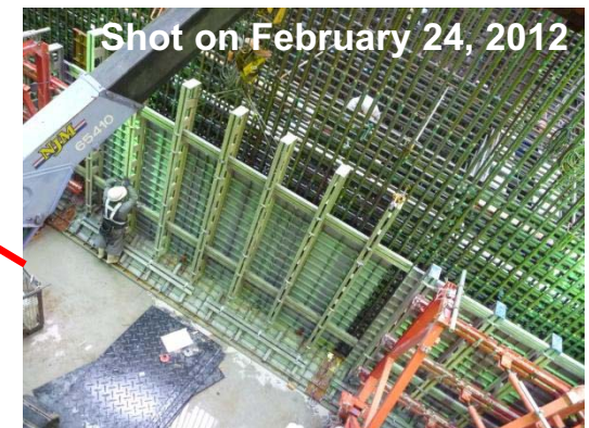
Placing steel enforcement for the bottom portion wall of the new pump room (No. 4)
