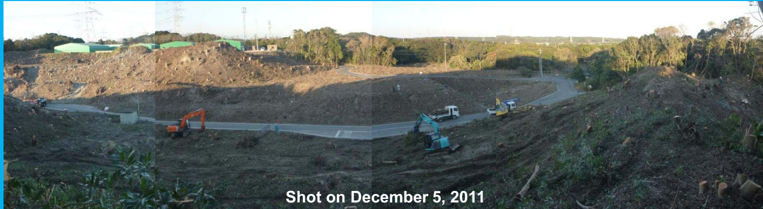
Preparation work of the high ground for the station site (T.P.+40 m) (four pictures are combined)
