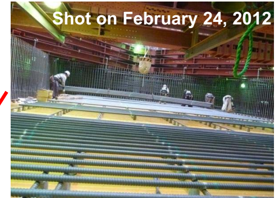
Placing steel enforcement for the wall portion of the first intermediate floor of the new pump room (No. 3)
